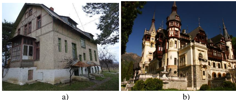
Figure 5. a) Traditional house with timber skeleton and masonry infill (only at 1st story and attic), from Chiojdeni, Vrancea county; b) Peleş Castel from Sinaia, Prahova county
